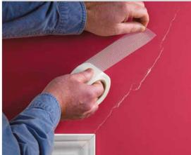
Ideal for hole repairs and crack reinforcement on all types of walls.
