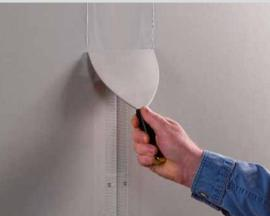
Self-adhesive tape saves time by eliminating the need for a pre-bedding coat.
